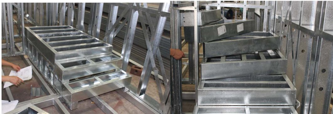
Set the stair
