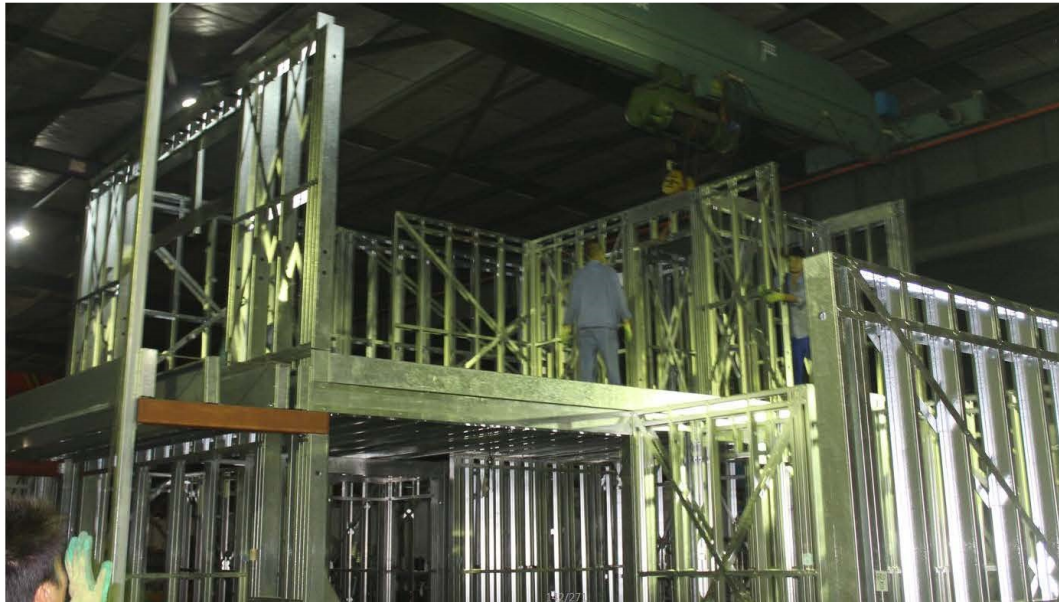
Set the ground floor wall
