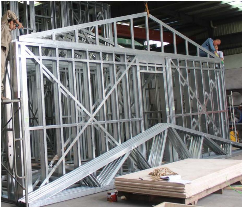
Set the Ground floor wall
