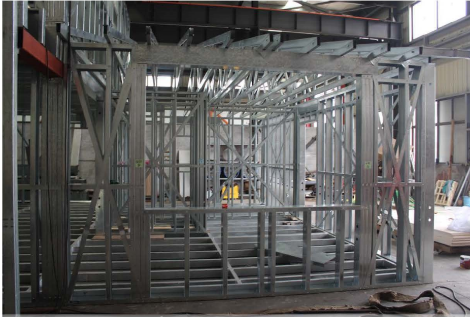
Set the ground floor wall
